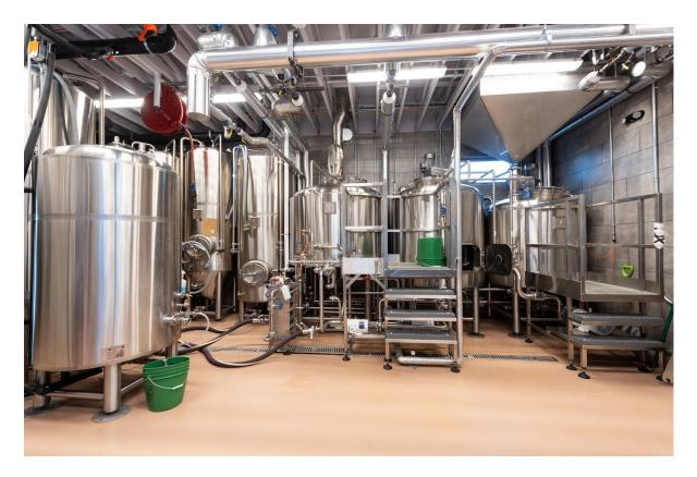
The RiNo Brewhouse is outfitted with a completely customized system to leverage every square foot of the confined space. Complete with six fermenters, a dedicated hot liquor tank, and a custom-built hop back, the system was designed to handle a myriad of styles and brewing techniques.
